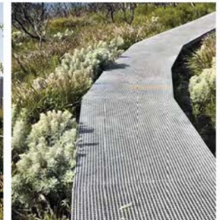
Raised platforms and walkways
